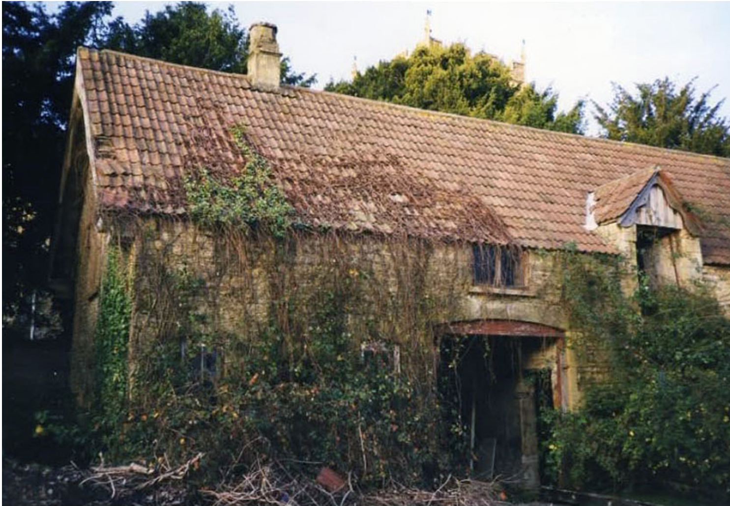
Photo 7 The Barns from Canon Court Farm
